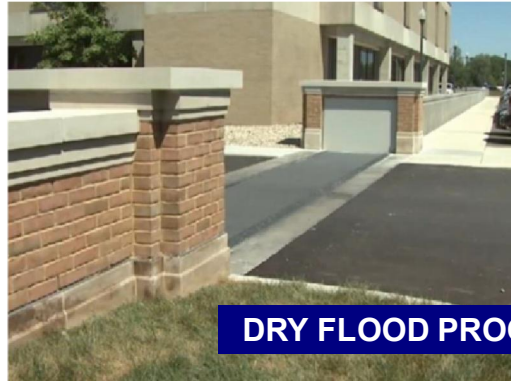
Use of flood barriers, installed at the entrance of the buildings (SHIELDING)
