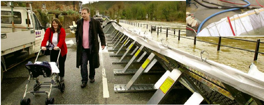
Flood barriers along riverbanks or crossing a street (SHIELDING)
