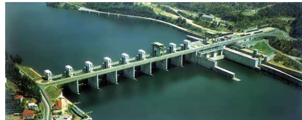
Example of run-of-river dam: Crestuma dam
