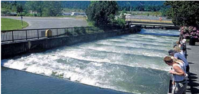
Fish ladder at Bonneville dam (USA)
