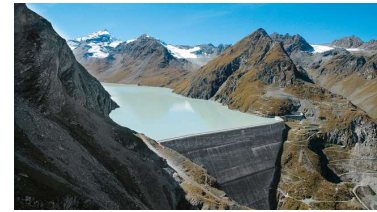
Grand Dixence dam (Switzerland)
