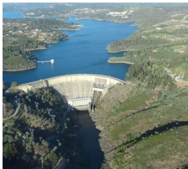
Spillway and water uptake tower at Castelo de Bode reservoir.
