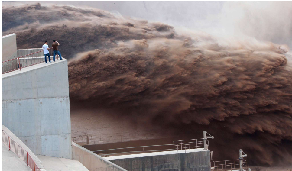
Discharge at Xiaolangdi dam (Yellow river, China), in July 2012
