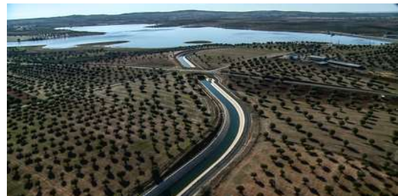
Alqueva irrigation channel
