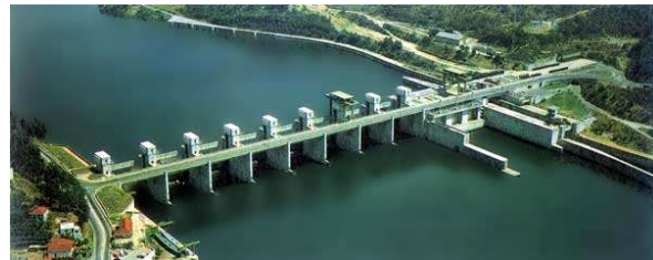
Example of run-of-river dam: Crestuma dam
