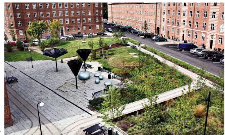
ΔΠΘ ΗΜΕΡΙΔΑ 23 ΟΚ Figure 28. Tansinge Plads - square and a water retention basin, designed to hold back
