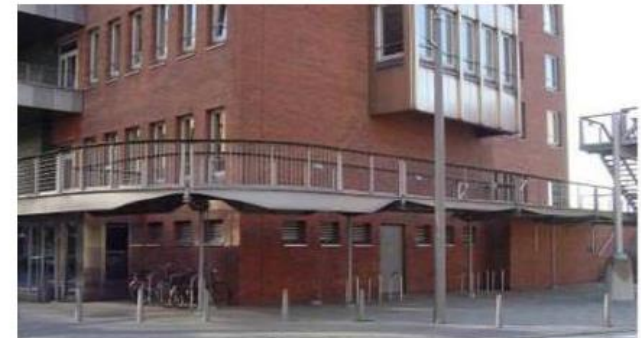
Figure 5.12 Example of dry proofing Hamburg, Germany
