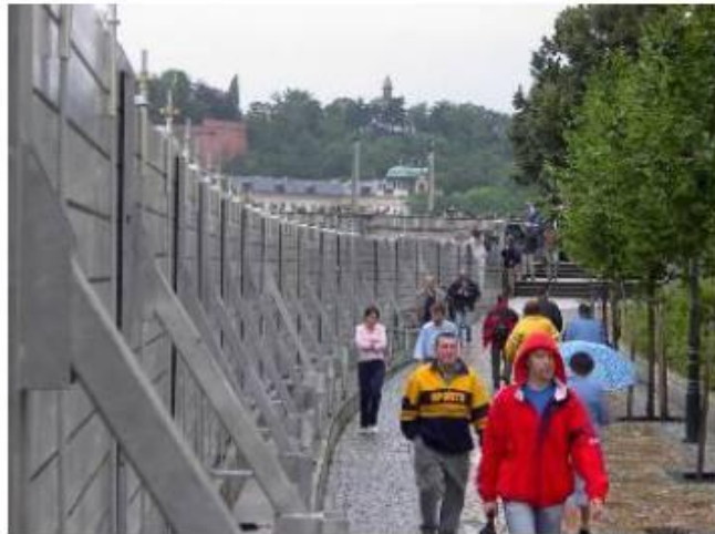
Figure 5.17 Temporary barriers in Prague, Czech Republic Source: VRV company, 2007
