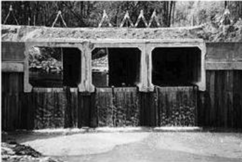
Culverts of rectangular c/s
