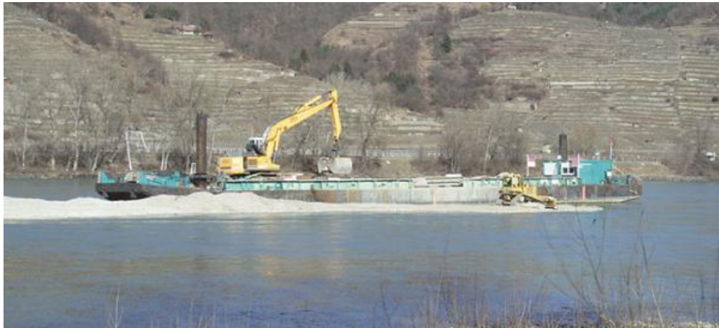
Figure 8: Artificial island building at the Danube River
